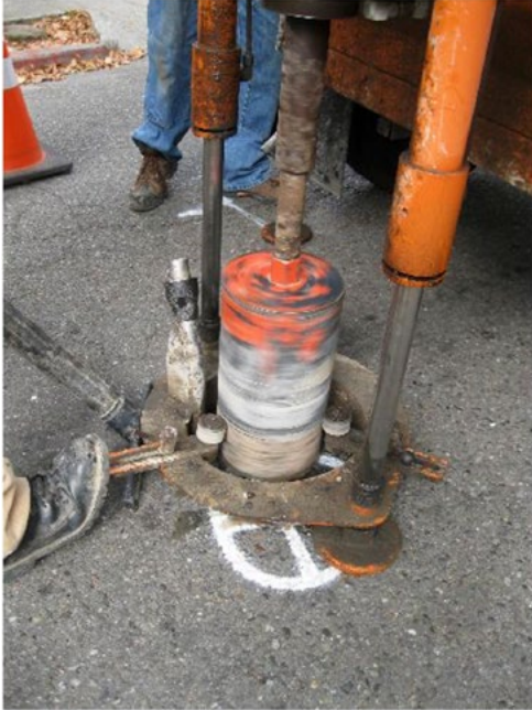
a. Core barrel.
