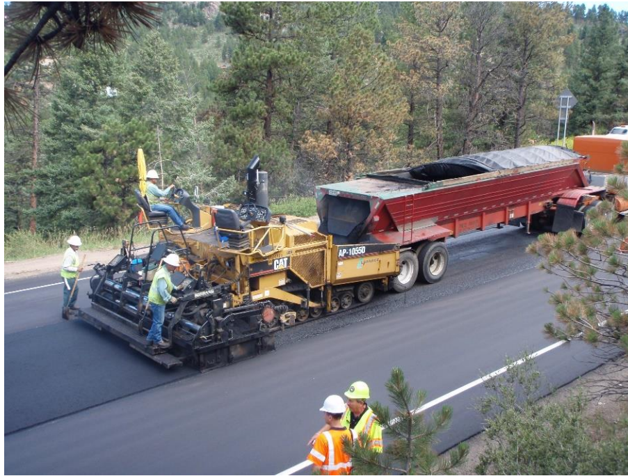
Figure 75. Live-Bottom Truck
