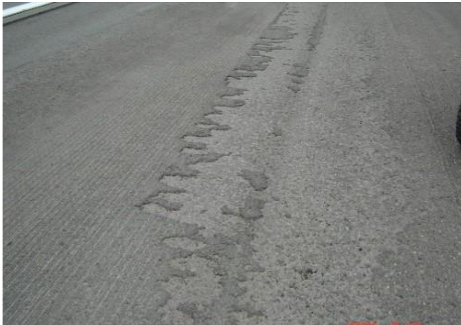
Figure 15. Raveled Asphalt Pavement Surface
