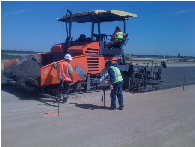
Figure 105. Stringline on an Airfield Project
