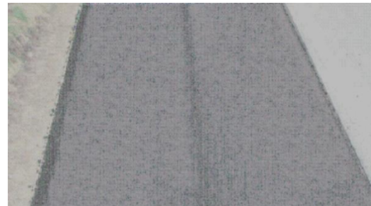
Figure 152. Examples of Centerline Segregation
