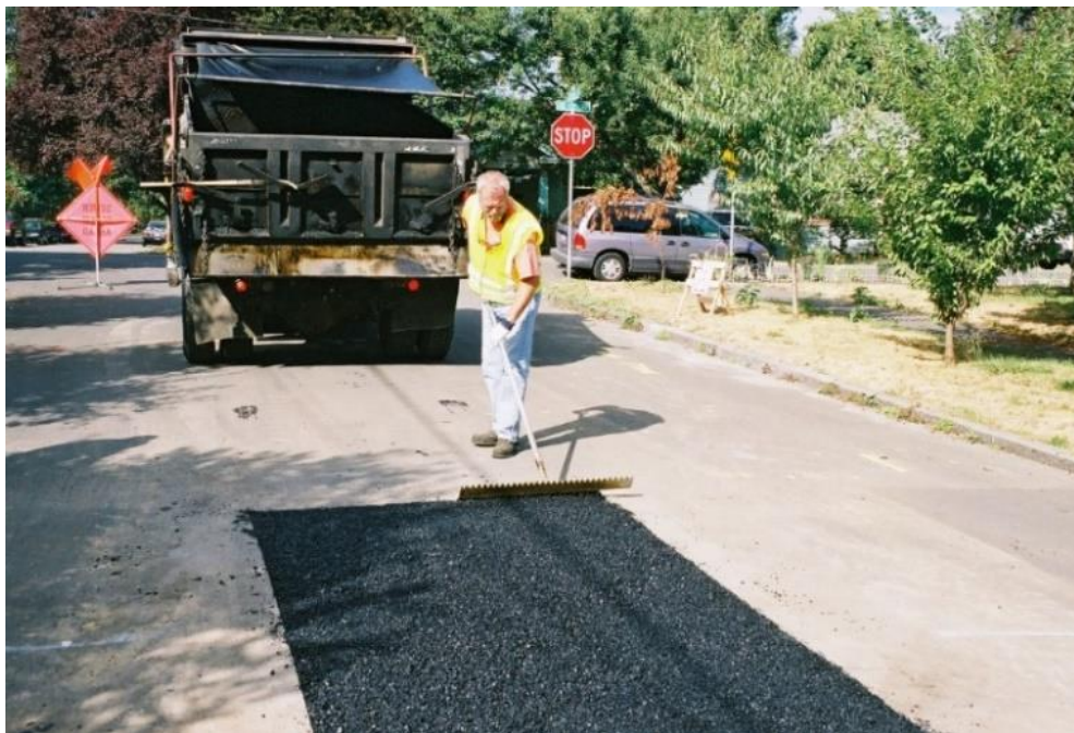
Figure 57. Material Placed in Localized Patch
