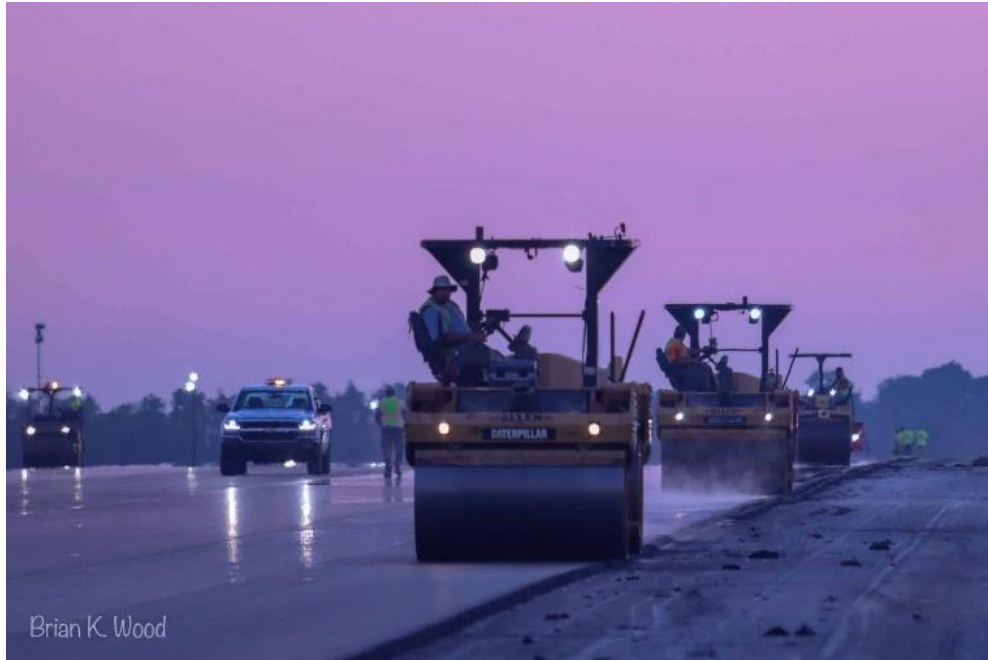
Figure 1. Roller Train Ensuring Compaction on a Runway Project
