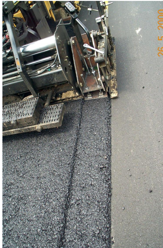
Figure 134. Notched-Wedge Device that Forms and Compacts through Screed Vibration
