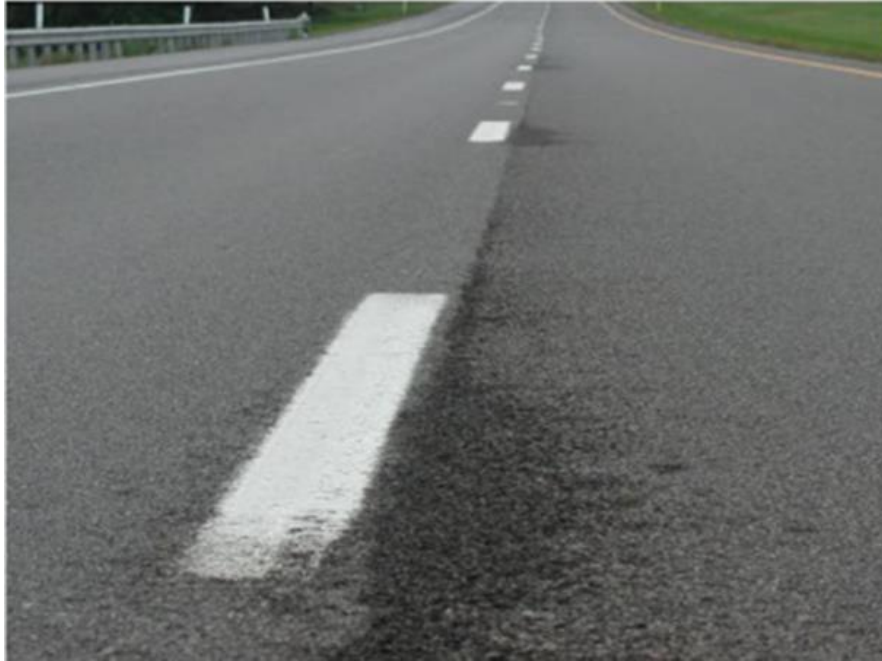
Figure 166. Poor Longitudinal Joint Due to Unsatisfactory Construction
