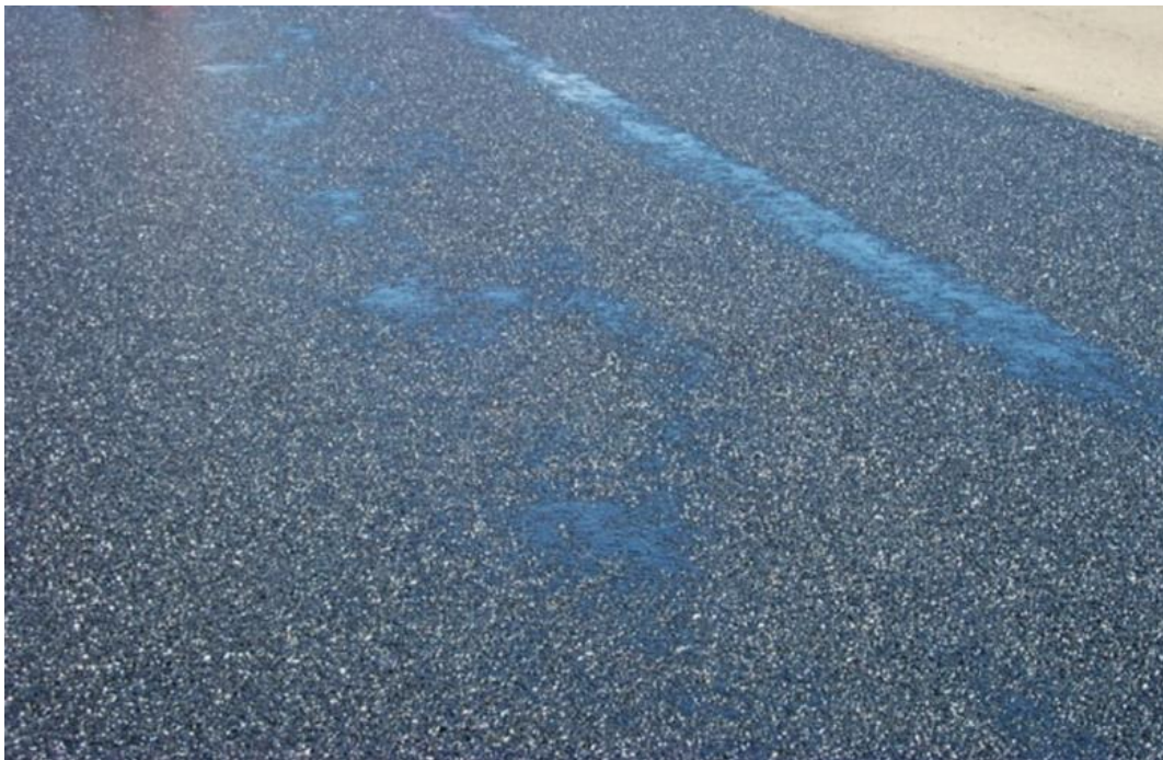
Figure 172. Fat Spot Caused by Localized Excess Asphalt
