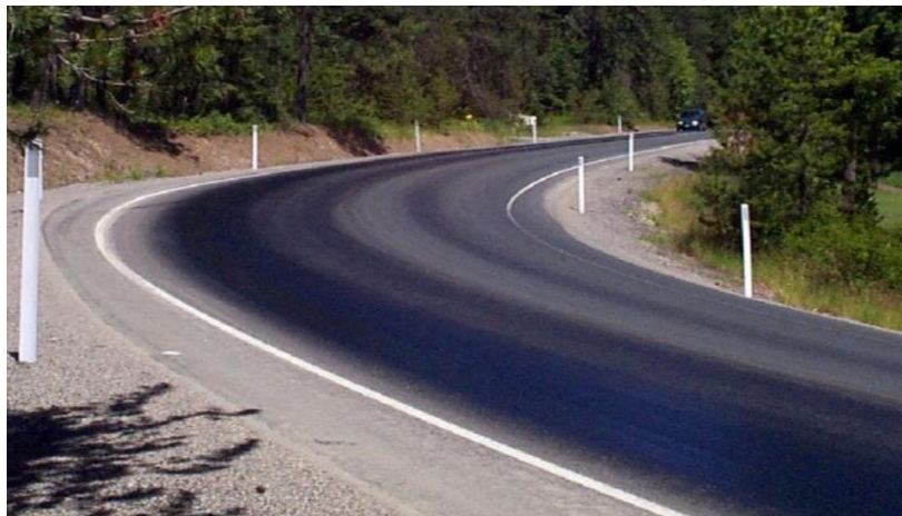
Figure 171. Asphalt Bleeding in the Travel Lane
