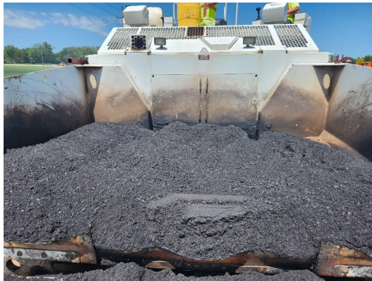
Figure 81. Paver Hopper Between Loads
