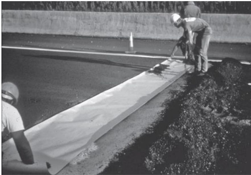
Figure 126. Placement of Kraft Paper Bond Breaker on Transverse Joint
