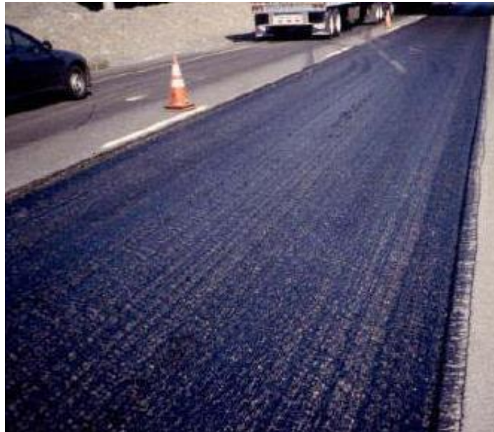
Figure 62. Tack Coat on a Milled Surface
