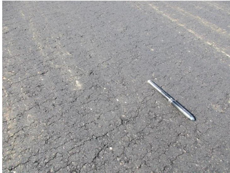
Figure 168. Hairline Cracks Caused by Roller Checking
