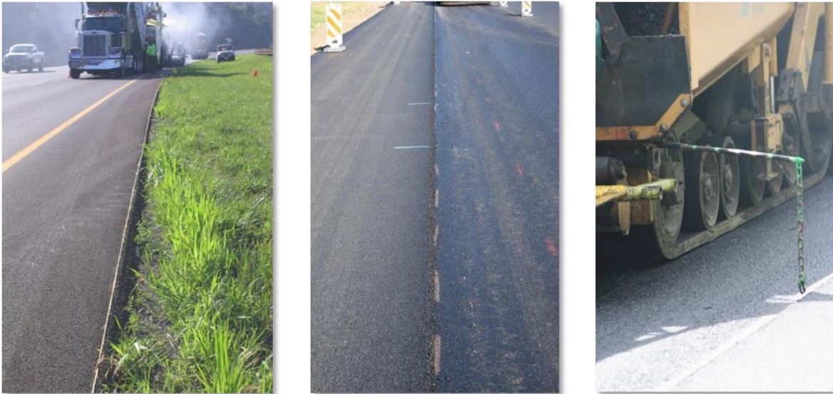
Figure 128. Paving in a Straight Line with Stringline, Skip Paint, and Guide on Paver
