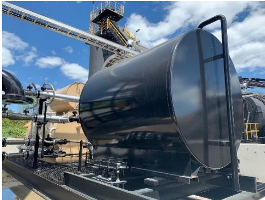
Figure 44. Stationary Asphalt Binder Calibration Tank
