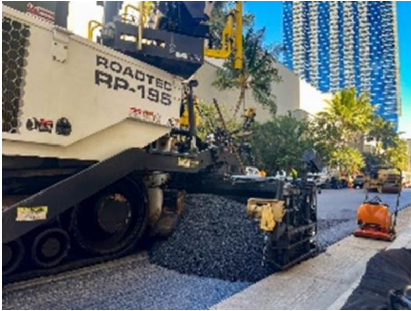
Figure 150. Improper Auger and Tunnel Extensions Cause Segregation
