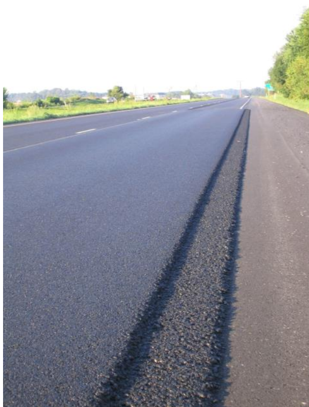
Figure 133. Notched-Wedge Joint with Taper at Top and Bottom of Wedge
