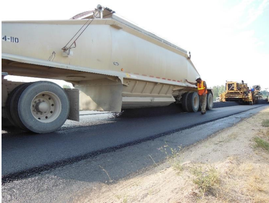
Figure 74. Bottom-Dump Truck
