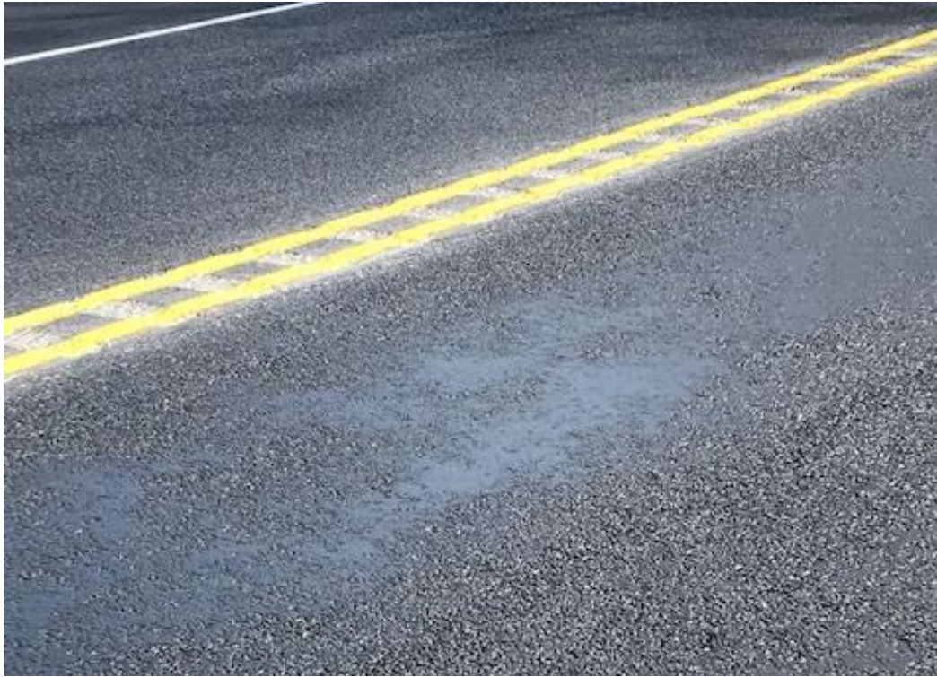
Figure 173. Fat Spot Caused by Fuel Oil Spill Prior to Overlay Construction
