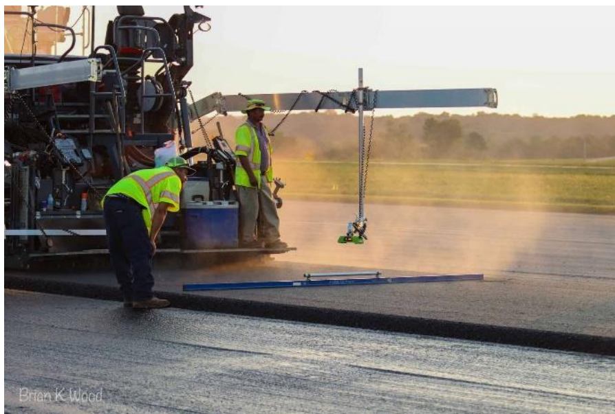
Figure 103. Over-the-Screed Grade Sensor and Cross-Slope Checking
