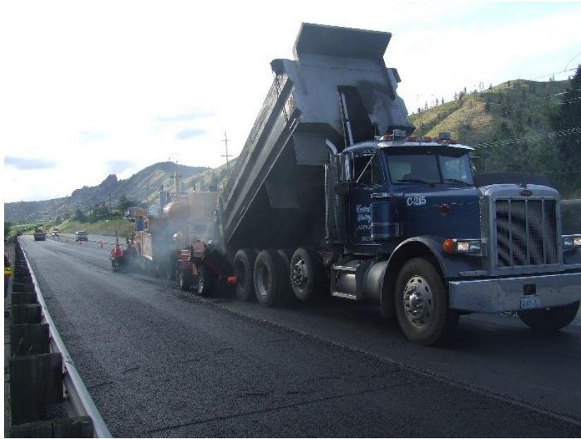
Figure 73. End-Dump Truck
