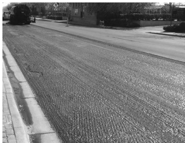
Figure 70. Tack Coat Application
