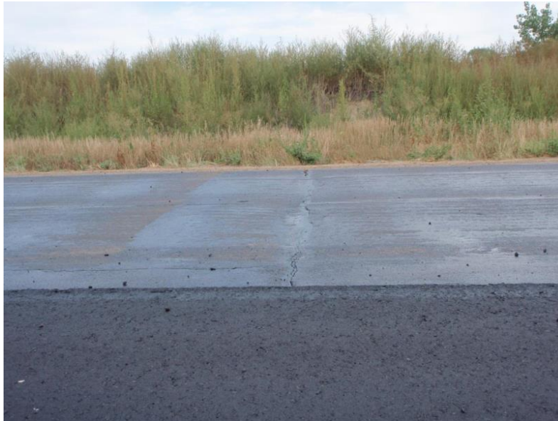
Figure 64. Non-Uniform Application of Tack Coat
