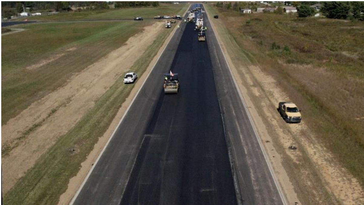
Figure 123. Longitudinal Joints on Airfield Runway
