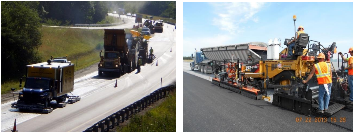
Figure 147. Joint Heaters: Self-Contained (left) and Paver-Mounted (right)
