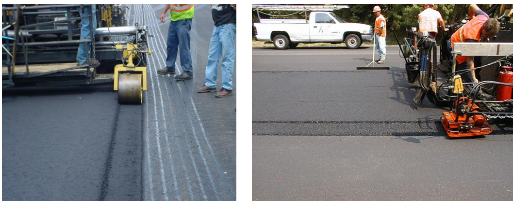
Figure 135. Two Devices for Compacting the Wedge of a Notched-Wedge Joint
