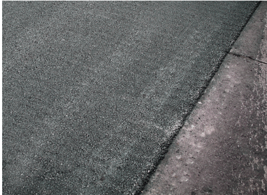
Figure 176. Washboard Marks Left by an Improperly Operated Vibratory Roller
