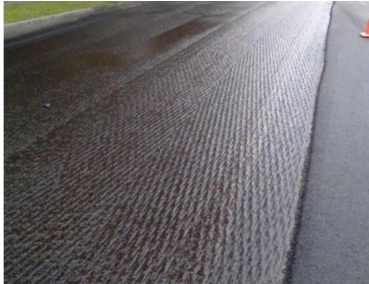
Figure 66. Uniform Application of Tack Coat
