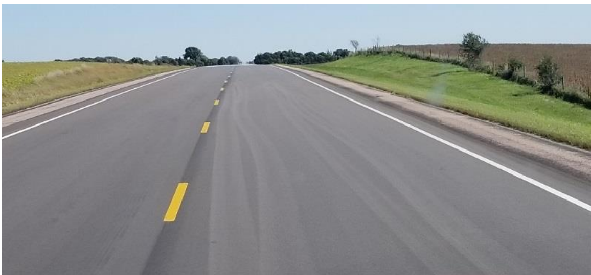
Figure 175. Pneumatic Roller Shadows in a New Asphalt Pavement
