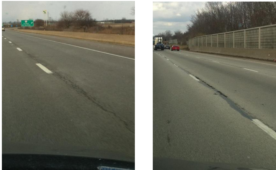
Figure 124. Premature Deterioration of Longitudinal Joints
