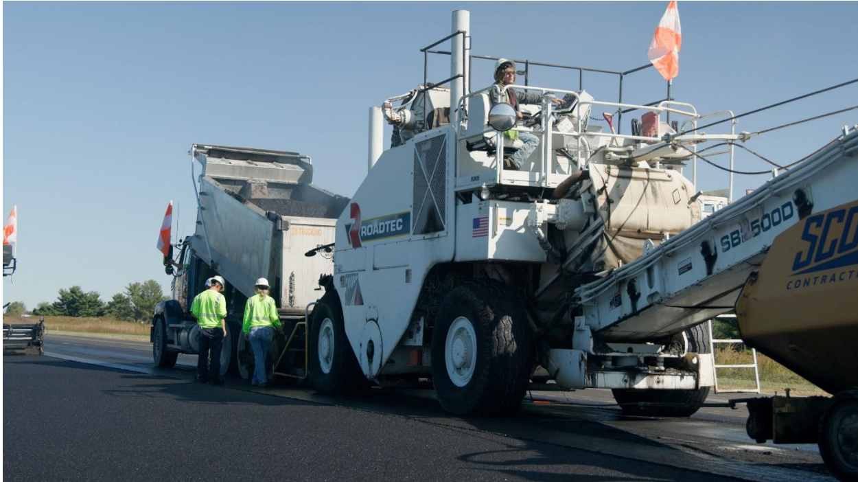
Figure 78. Material Transfer Vehicle
