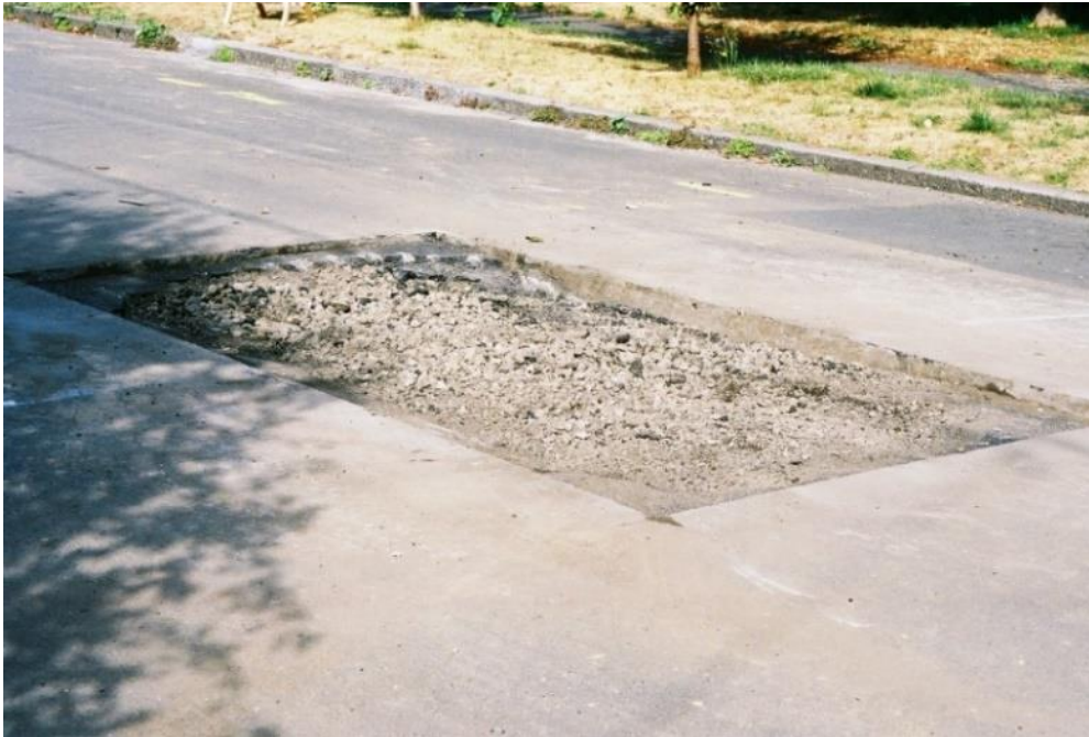
Figure 56. Existing Material Removed Prior to Patching
