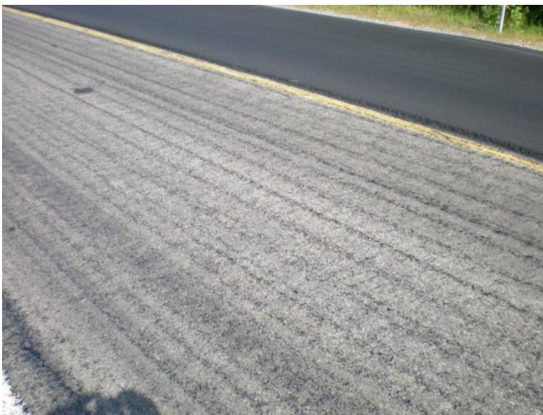
Figure 65. Non-Uniform Application of Tack Coat
