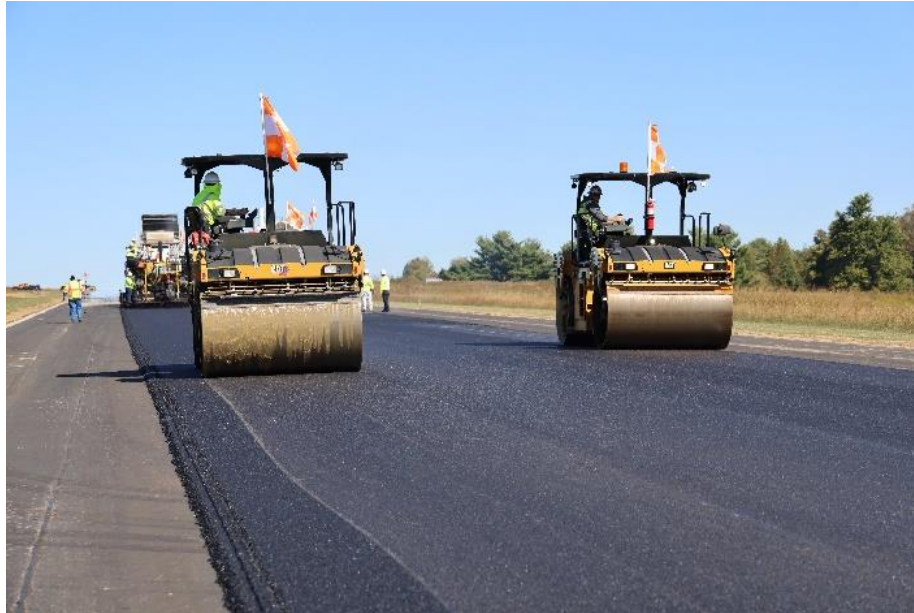
Figure 122. Breakdown Rolling with Two Vibratory Rollers
