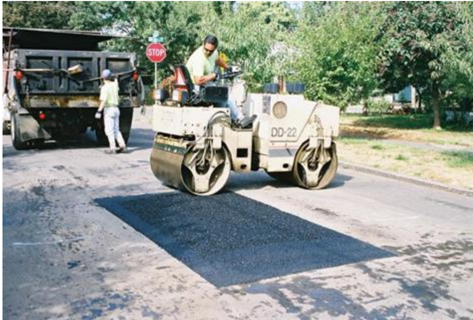
Figure 58. Compaction of Patch
