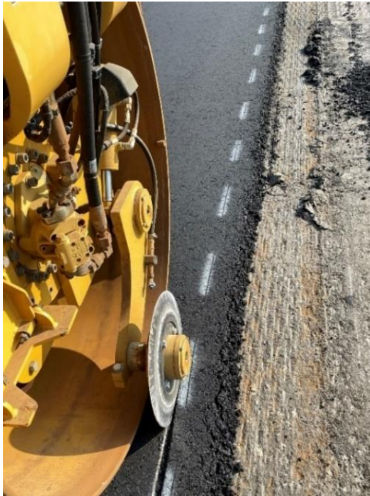
Figure 137. Cutting Wheel Mounted on a Roller
