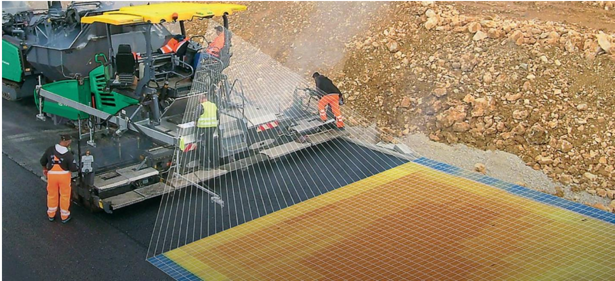
Figure 159. Paver Equipped with an Automated Infrared Scanner
