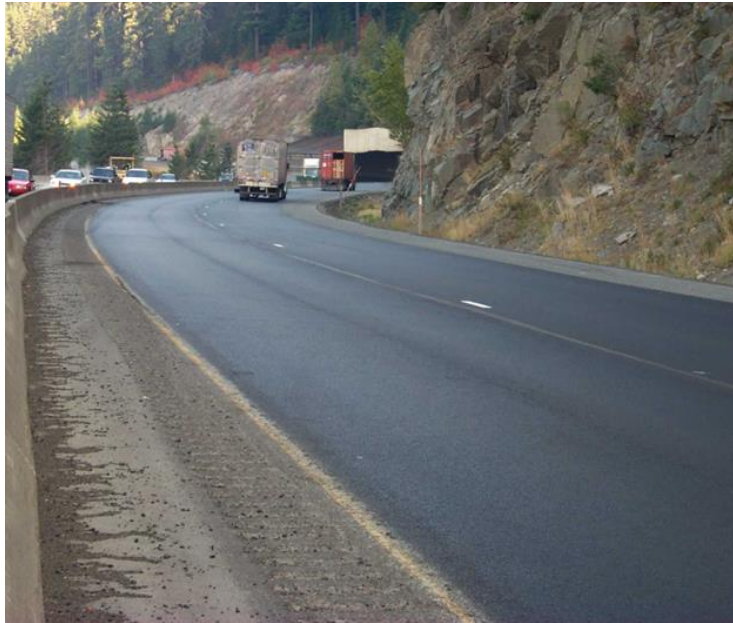
Figure 155. Example of Half-Width Mat Segregation
