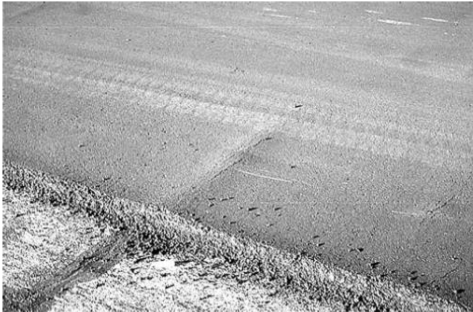
Figure 59. Bump Caused by Excessive Use of Crack Sealant
