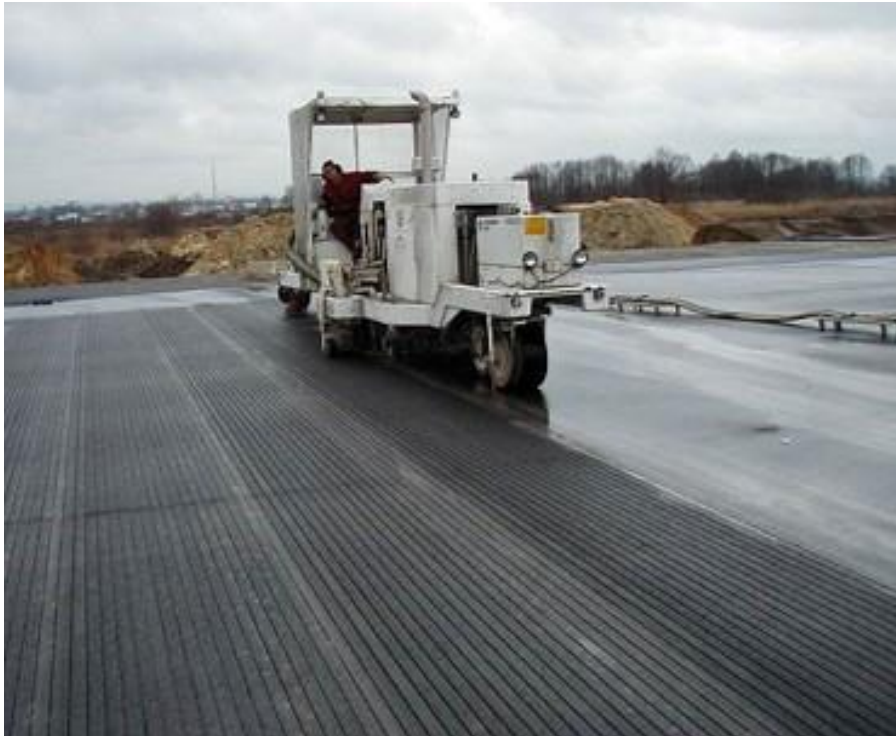
Figure 19. Grooving an Airfield Runway
