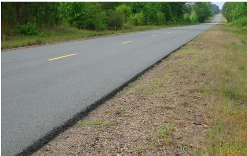
Figure 1: Picture taken in 2001 of LA 464 with plain RAP shoulders and typical shoulder drop-off (courtesy James Winford, Jr, PhD, PE)
