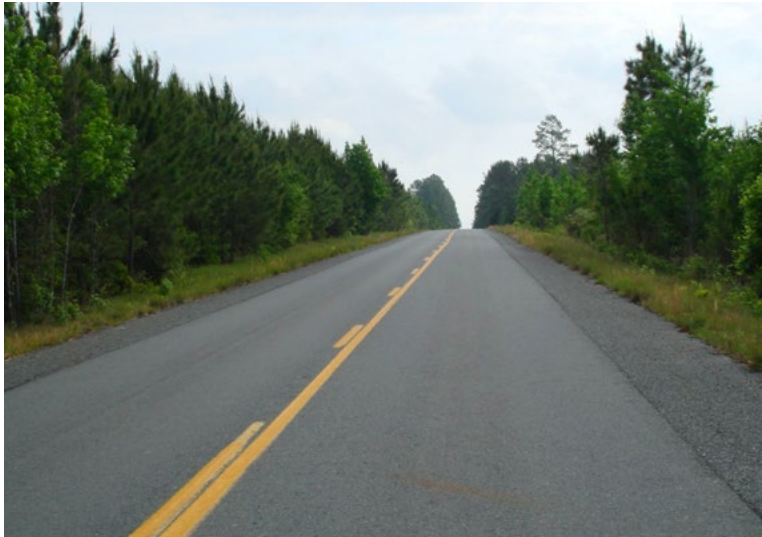
Figures 2 and 3: Pictures taken in 1999 of LA 464 (left) and Calcasieu Parish (right) using 'Hot RAP' on shoulders (courtesy James Winford, Jr, PhD, PE)
