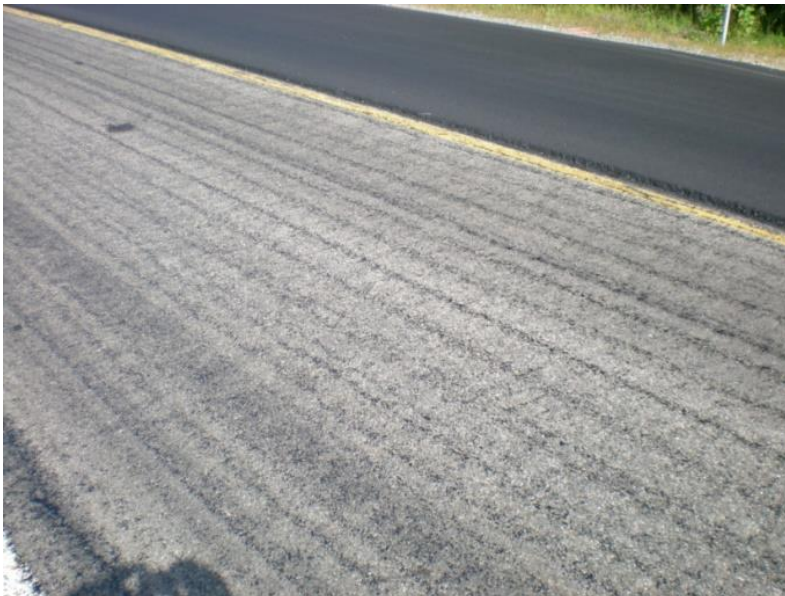
Figure 65. Non-Uniform Application of Tack Coat
