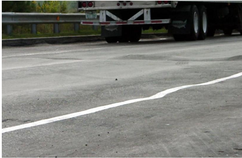
Figure 169. Shoving Due to Unsatisfactory Mix
