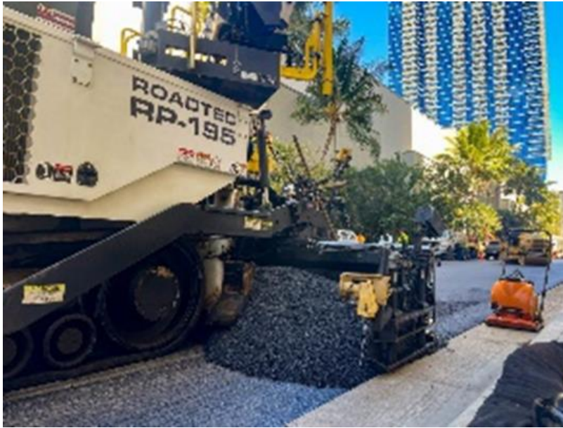
Figure 150. Improper Auger and Tunnel Extensions Cause Segregation
