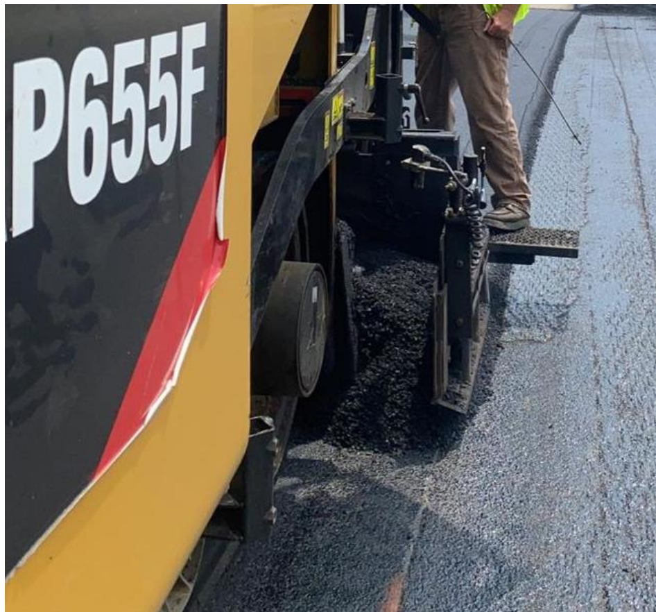
Figure 132. Poor Practice—End Gate Not Set to Be Seated on Existing Surface
