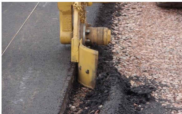
Figure 139. Kick-Out Plate Aids in Removing the Cutback Mix
