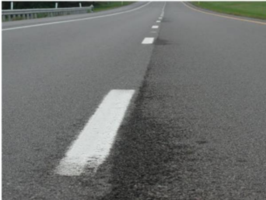
Figure 166. Poor Longitudinal Joint Due to Unsatisfactory Construction
