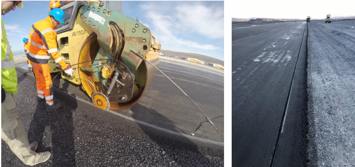
Figure 140. Stringline, Paint, and a Mounted Guide Allow Straight Cutting
