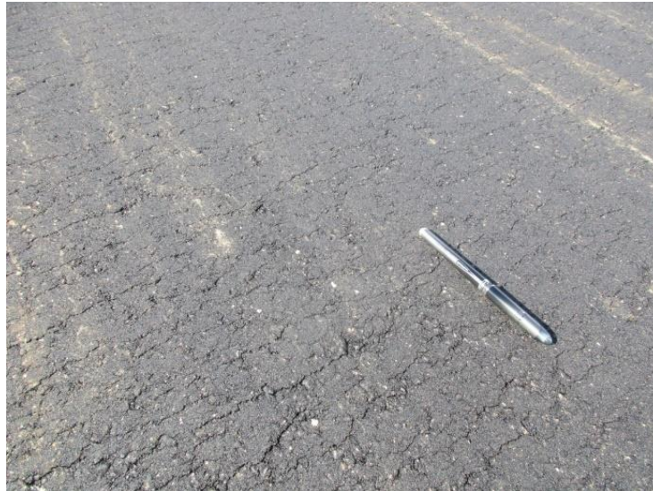
Figure 168. Hairline Cracks Caused by Roller Checking
