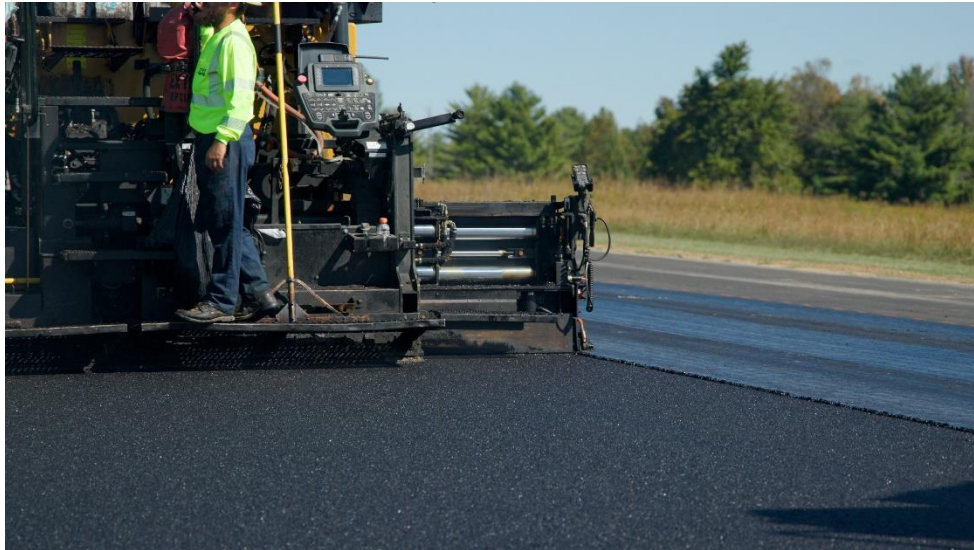
Figure 93. Extendable Screed Paver
