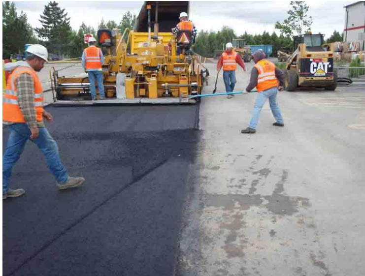
Figure 145. Improper Broadcasting and Luting across the LJ
