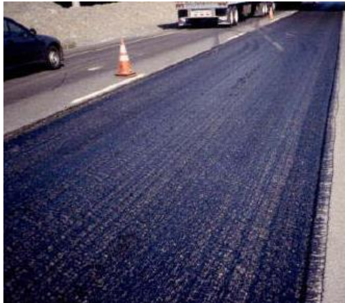
Figure 62. Tack Coat on a Milled Surface
