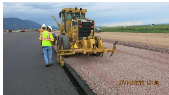
Figure 139. Kick-Out Plate Aids in Removing the Cutback Mix
