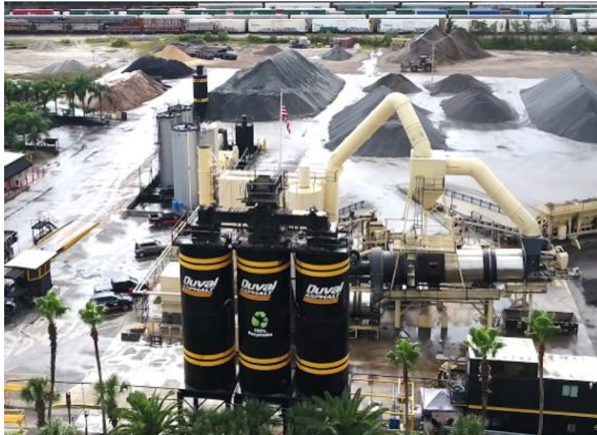
Figure 51. Insulated Storage Silos
