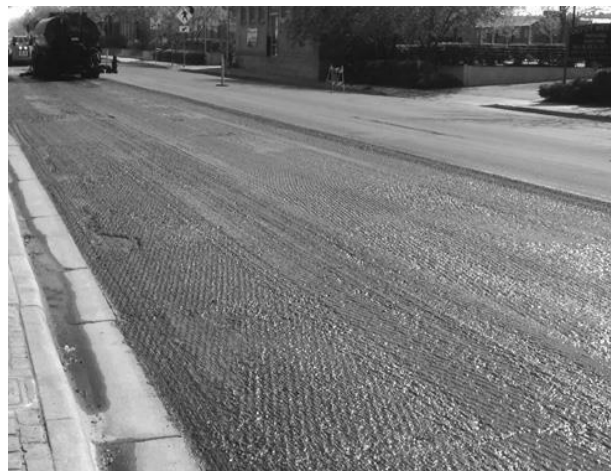
Figure 70. Tack Coat Application
