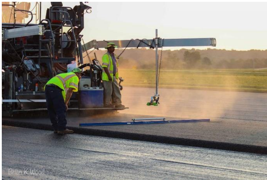
Figure 103. Over-the-Screed Grade Sensor and Cross-Slope Checking
