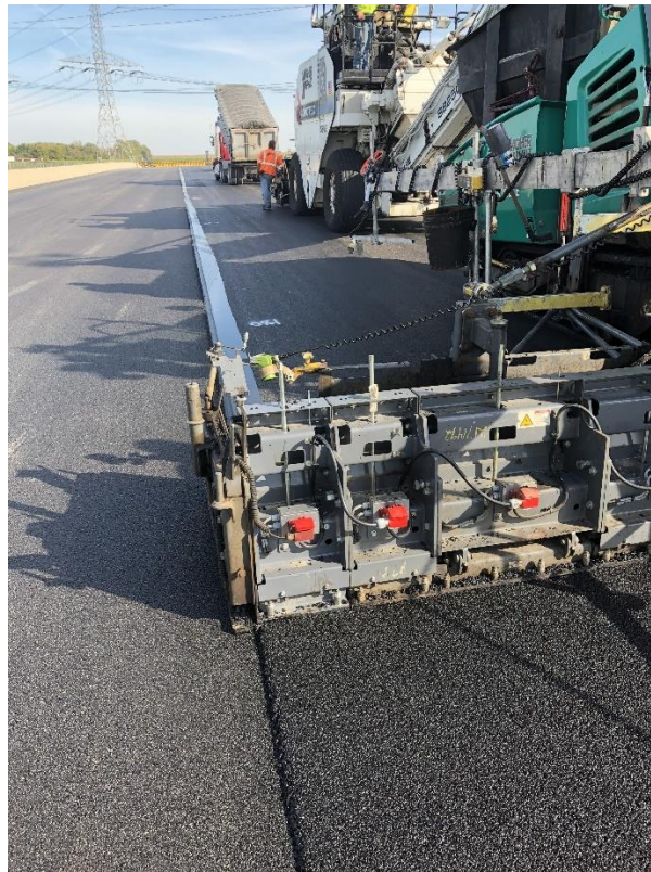
Figure 92. Fixed-Width Screed with Vibratory Bolt-On Extensions
