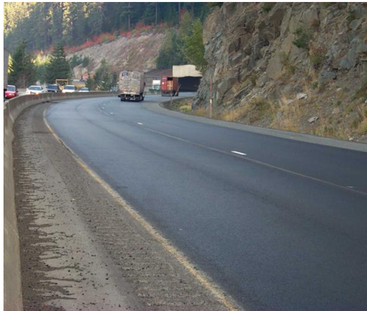
Figure 155. Example of Half-Width Mat Segregation
