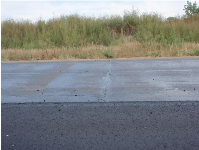
Figure 64. Non-Uniform Application of Tack Coat
