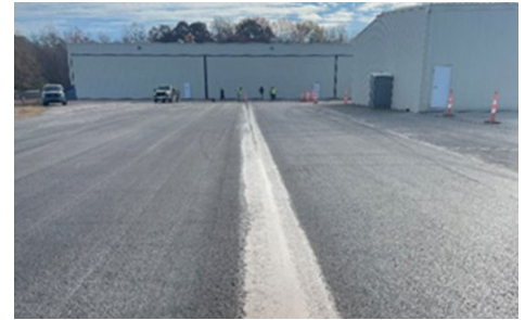
RPE application on the butt joint of a crossover taxiway.
