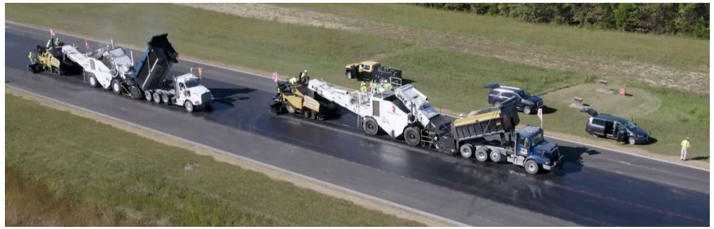
Crews pave a longitudinal joint on a runway in Leitchfield, KY.
