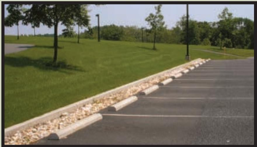
**Figure 6 – In the event that the surface is repaved, an unpaved stone edge will still allow stormwater to reach the stone bed.**
