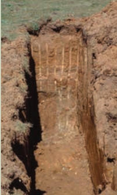
**Figure 7 – Excavating a “deep hole” with a backhoe allows field investigation of the soils prior to construction.**
