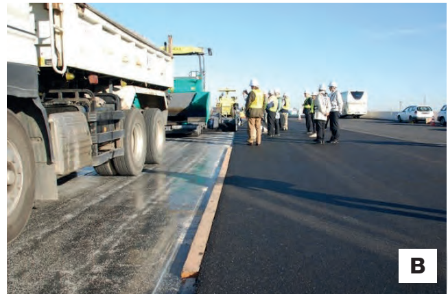
Figure 3-2. A) Technician checking mix temperature of every truck load before dumping into the paver; B) Lumber used along previously placed mat to protect the vertical edge as haul trucks move in and out of paving lane; C) Mix is transferred from the haul truck directly into the paver hopper; and D) Paver screed and mat.
