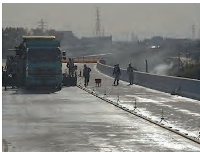
Figure 3-4. Left: Paving on the Satte viaduct. Wooden forms are set for the unconfined edge. Right: After paving the wooden forms are still in place.
