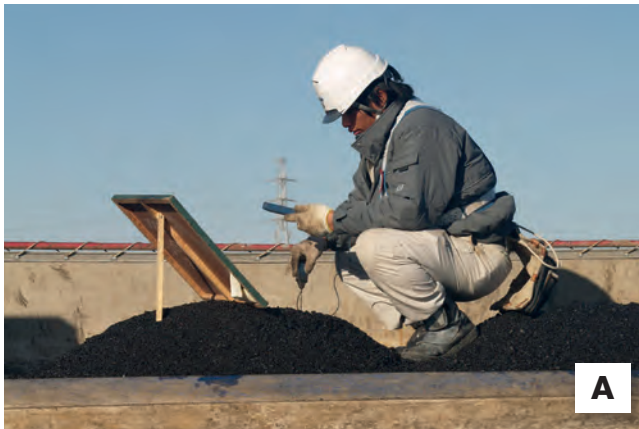
Figure 3-2. A) Technician checking mix temperature of every truck load before dumping into the paver; B) Lumber used along previously placed mat to protect the vertical edge as haul trucks move in and out of paving lane; C) Mix is transferred from the haul truck directly into the paver hopper; and D) Paver screed and mat.
