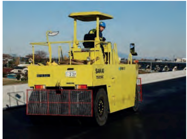
Figure 3-5. Left: A three-wheel roller was used for breakdown compaction. A pneumatic-tire roller is seen in the distance. Right: Pneumatic-tire roller used for intermediate compaction.
