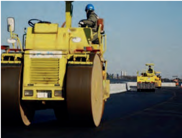
Figure 3-5. Left: A three-wheel roller was used for breakdown compaction. A pneumatic-tire roller is seen in the distance. Right: Pneumatic-tire roller used for intermediate compaction.
