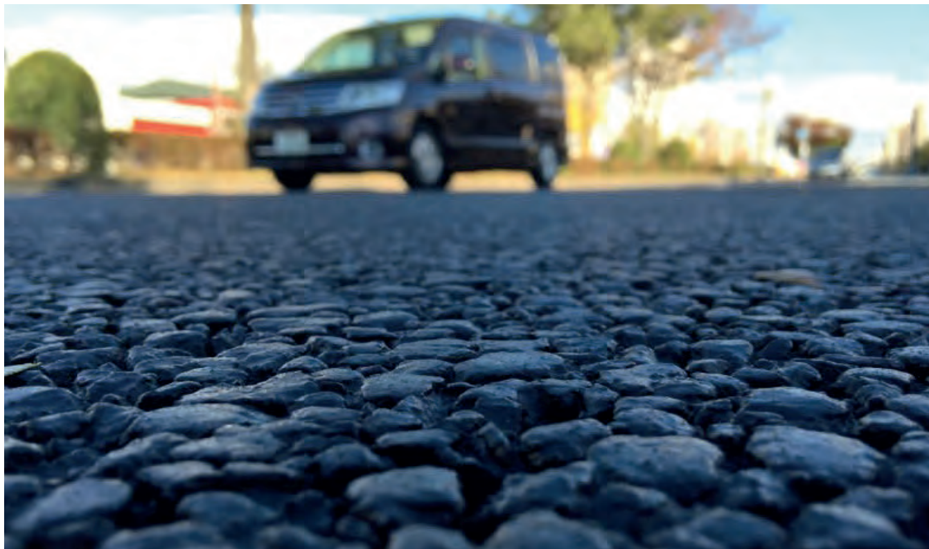
Figure 4-1. Recently constructed porous friction course in Kyōto
