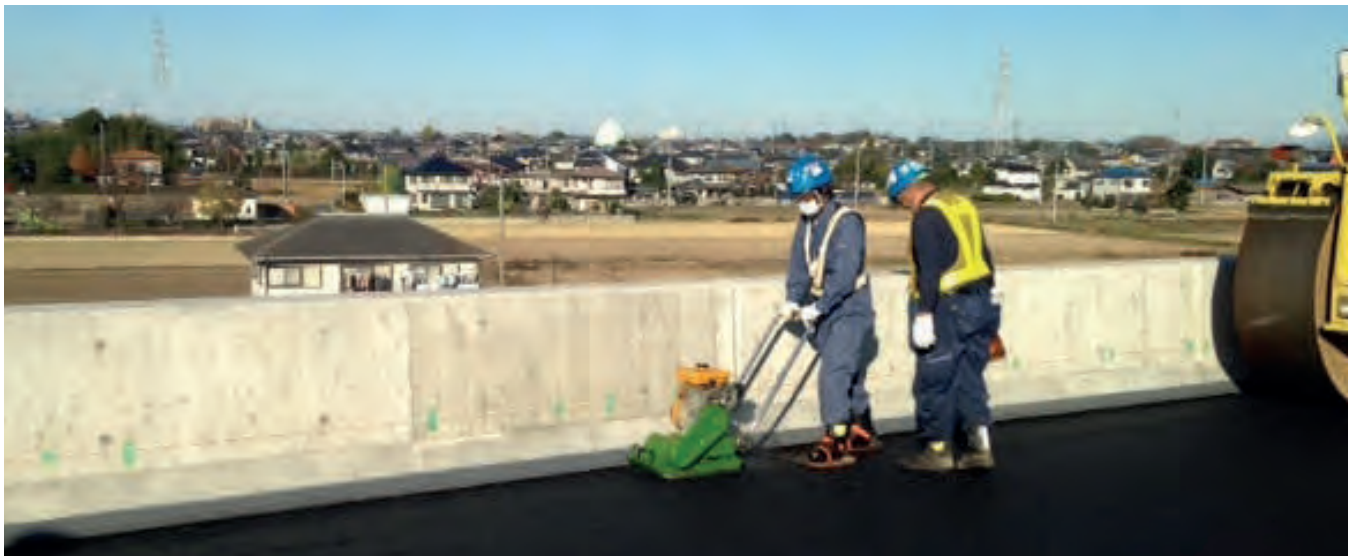
Figure 3-6. Compaction of the asphalt mix along the barrier wall with a vibratory plate compactor.
