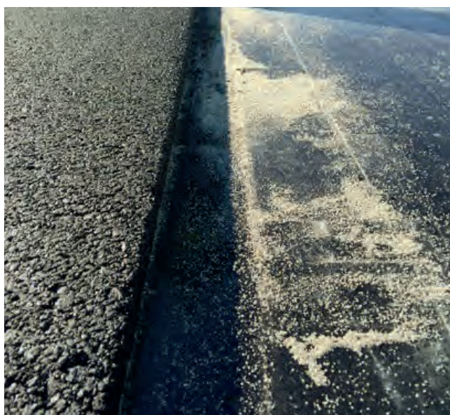
Figure 3-4. Left: Paving on the Satte viaduct. Wooden forms are set for the unconfined edge. Right: After paving the wooden forms are still in place.
