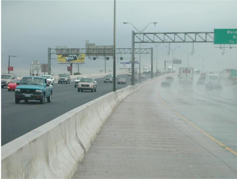
Figure 1. Vehicle tire spray driving with and without a PFC pavement (I-35, San Antonio)
