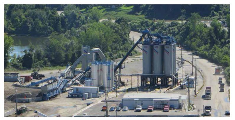
ated during the drying of aggregate, are captured by baghouse filters or similar controls and never released to the environment.
