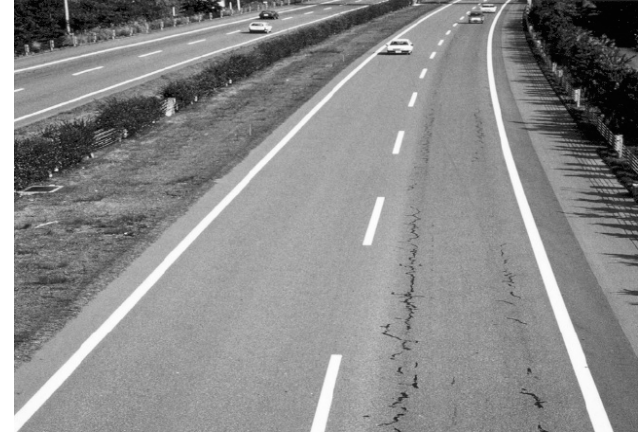
Top-down cracking
