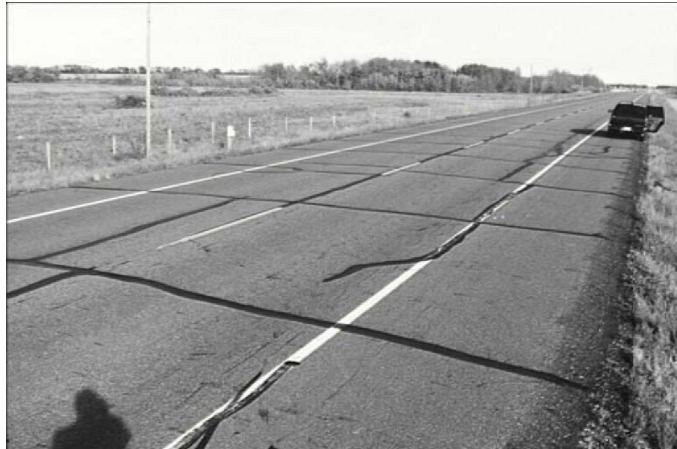
Transverse cracking
