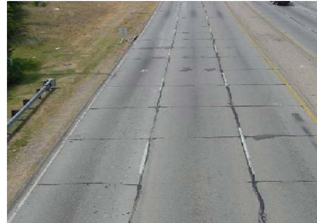
Reflection cracking
