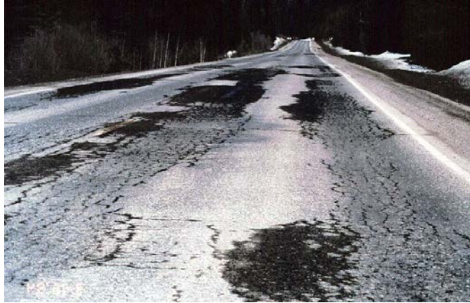
Bottom-up cracking
