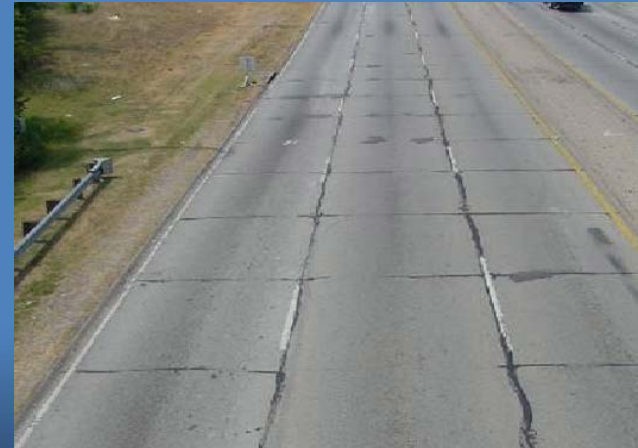
Reflection cracking
