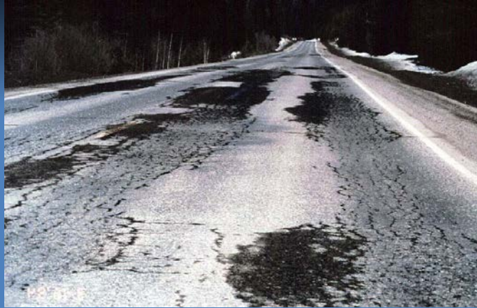
Bottom-up cracking
