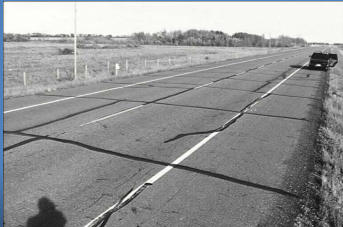
Transverse cracking
