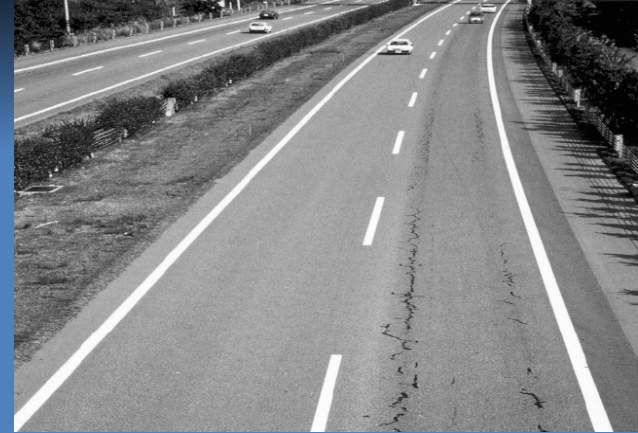
Top-down cracking
