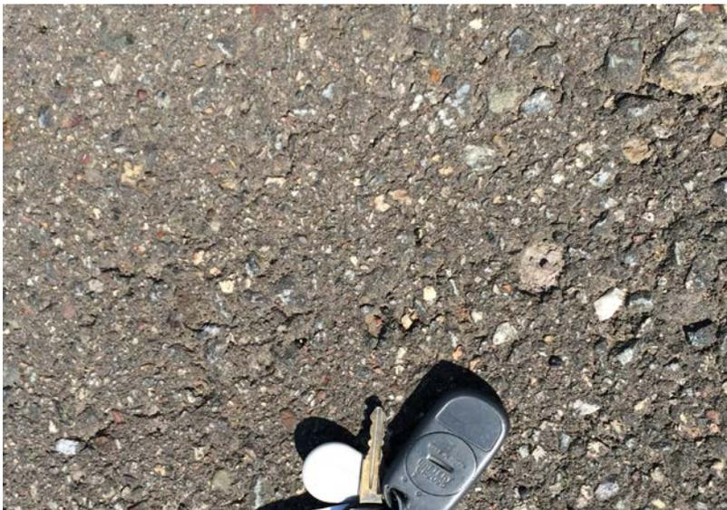
Figure 3: Example of Loss of mastic, raveling (3yr, WI I90/94)
