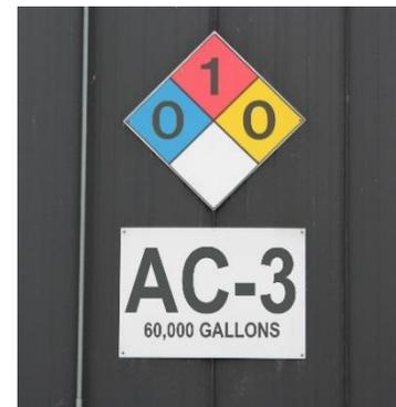
Similar labels may be required for fuel storage tanks, chemical additive tanks, or other liquid storage tanks. In addition, signage similar to "Caution: Hot" may be appropriate near any sampling or access point where there is potential for workers to contact hot surfaces or liquids.
